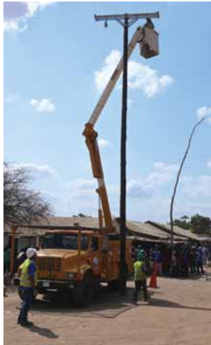
Pike workers install medium-voltage wire, which will supply electricity to Chamae Village for the first time.
