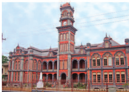
Restoration of the Queen's Royal College Building
