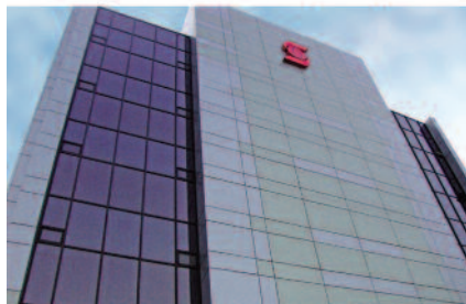
Scotia Centre - Exterior Renovation
